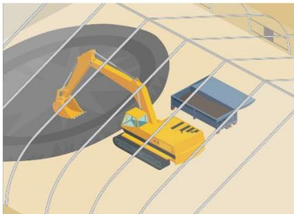
Excavated Pit F waste will be loaded into bins which will be sealed for transport while inside the tent
